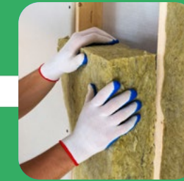
Insulation of Roof and External Walls
